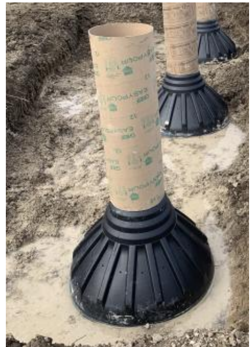
Diagram 3: Pre-molded pier forms
